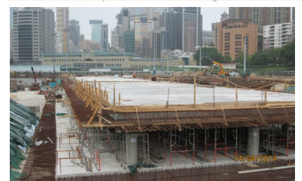
Section of top slab of the stormwater tank completed
