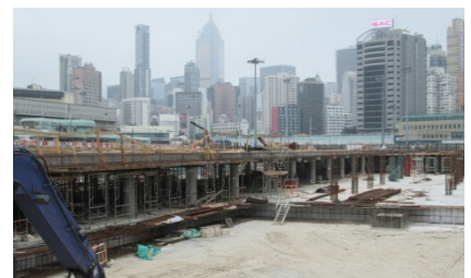
Excavation in progress for next section
