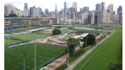
Excavation from Northeast corner of the recreation ground
